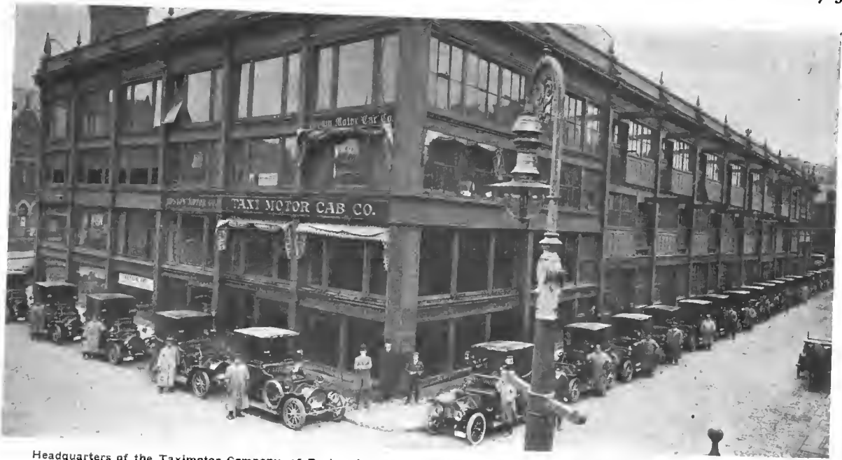
Headquarters of the Taximotor Company, of Boston, in the Motor Mart, Park Square, and its Equipment of Thomas Taxicabs.
